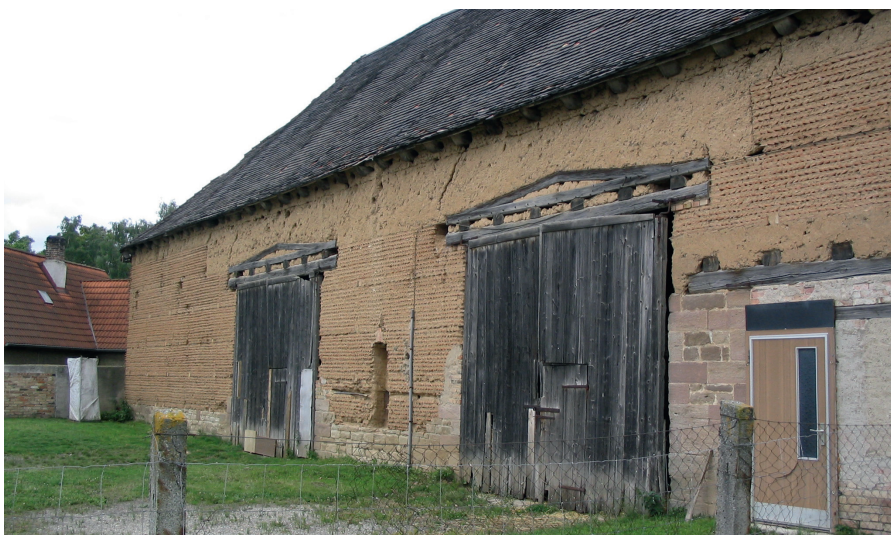
Fig. 10.23 : Rammed earth barn with weller earth sections over the en- trances in Jüdendorf/ Saxony-Anhalt, 2006
