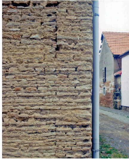
Fig. 10.24 a and b : Rows of embedded brick and tile visible on the surface of rammed earth walls
