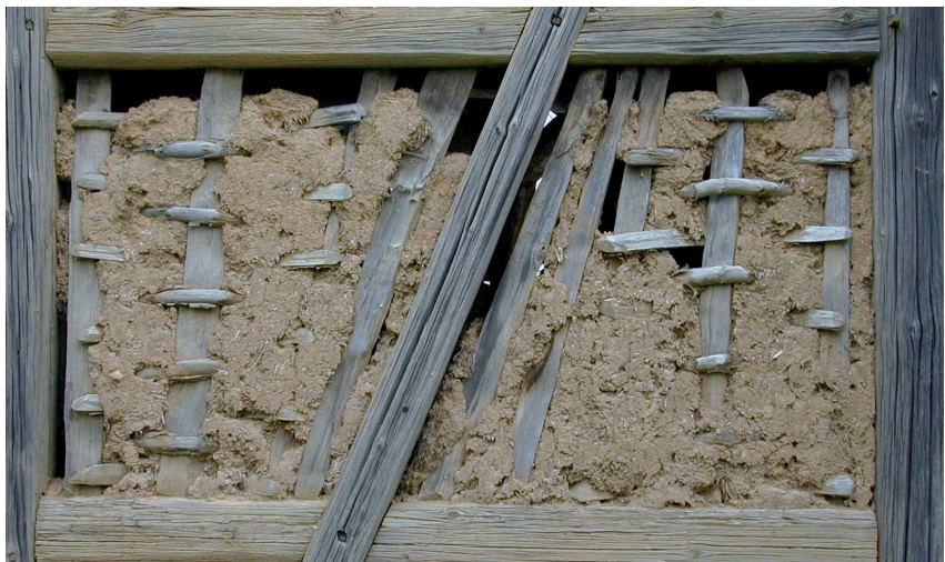
Fig. 10.49 : The panel of a timber-frame house in Saxony
